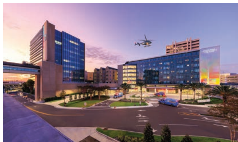
Wolfson Children’s Hospital, photo courtesy of Baptist Health
