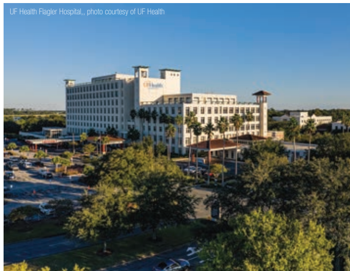
UF Health Flagler Hospital, photo courtesy of UF Health
